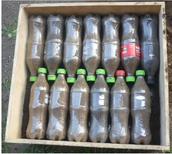
Figure 8. Placing the second layer of PET bottle.
