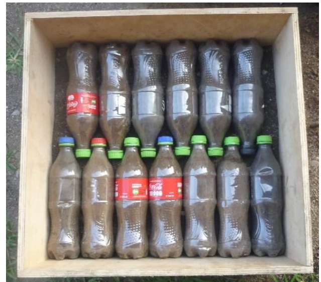
Picture 6. First layer of PET bottle filling with sand.
