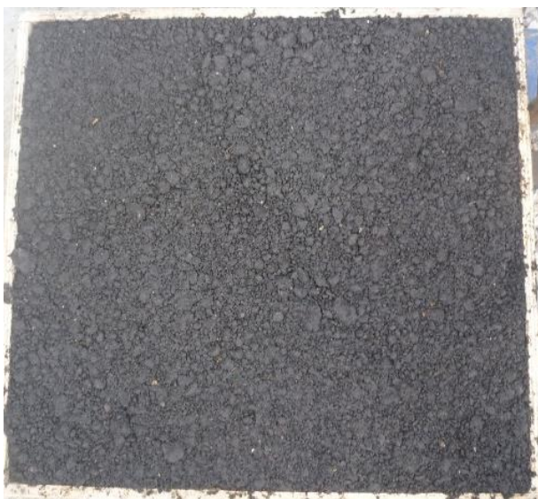
Figure 9. Placing the asphalt layer at the end of the pothole repair.
