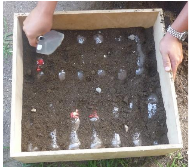
Picture 7. Filling the space between bottle with sand.
